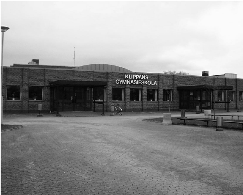
Figure 5.8 The school in Klippan.
